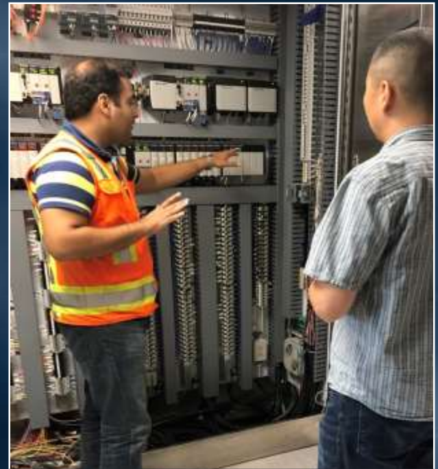
Control System Integration
