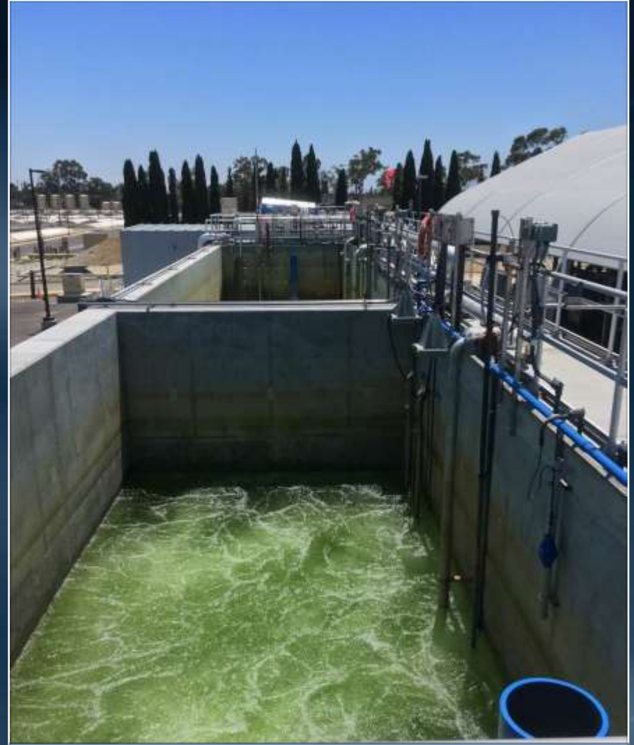
Aerobic Basin Preparation
