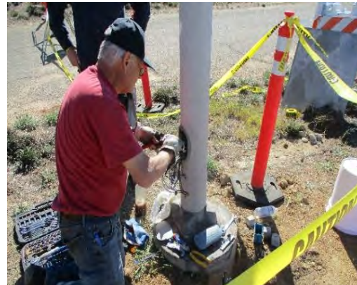
Staff excavating for new conduit (left) and performing circuit repairs (right)
