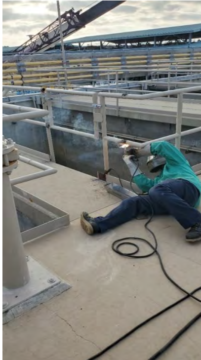
Staff welded new filter access gates into the existing filter perimeter railing at the Skinner plant
