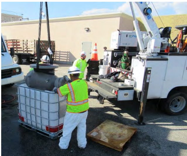
Staff disinfecting (left) and preparing to install (right) a new valve at the Santa Monica Feeder
