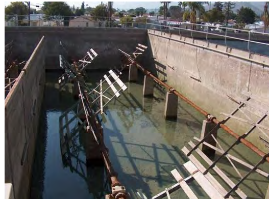
Staff performing maintenance on flocculator paddle drive chain at Weymouth plant
