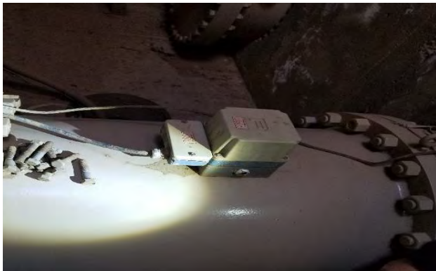
Existing meter (left) and staff preparing to replace flow meter (right) at EM-04 service connection
