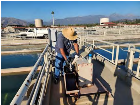
Staff performing maintenance on flocculator paddle drive chain at Weymouth plant
