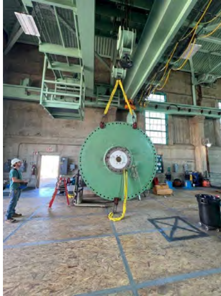
Staff inspected and installed discharge valve headcover at the CRA
