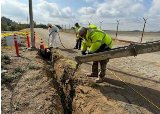
Staff placing electrical encasement
