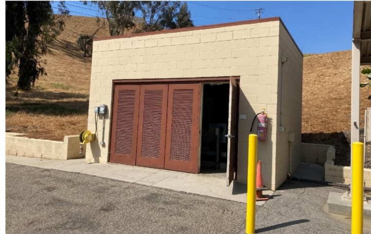
Photograph 2. Backup Generator Enclosure
