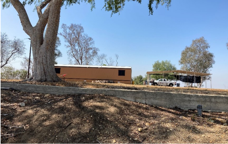
Photograph 1. Construction Trailer Staging Area
