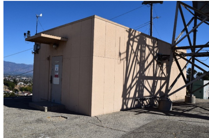
Photograph 4. Building at Communications Site
