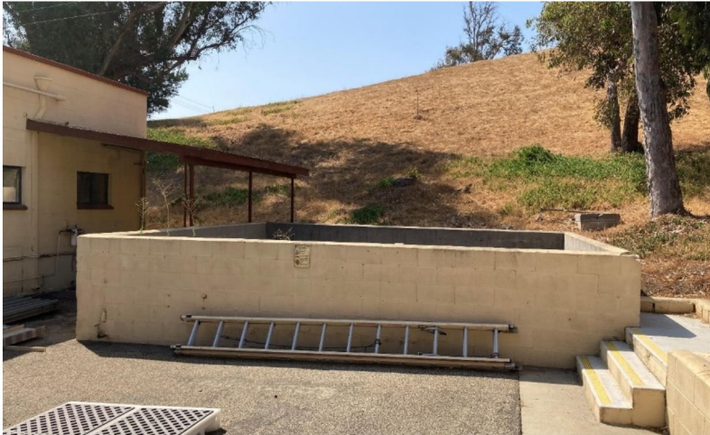
Photograph 1. Former Caustic Soda Structure
