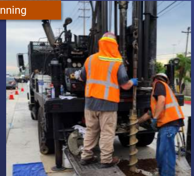
Geotechnical Borings
